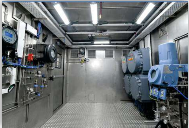
Analyzer Shelter for Natural Gas Processing Plant
