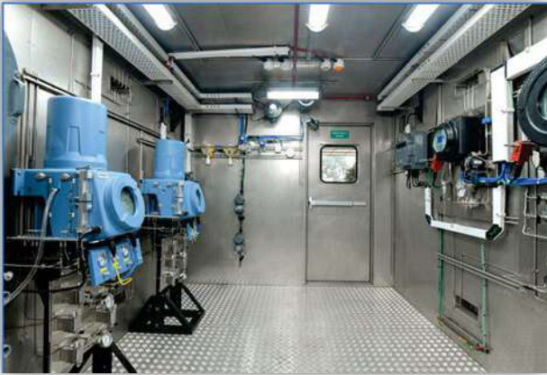
Analyzer Shelter for Natural Gas Processing Plant
